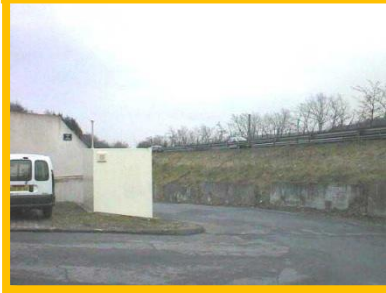
Station fixe Trafic Rive de Gier_A47
